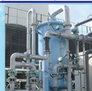
Removing Ferrous and Manganese filtration system
