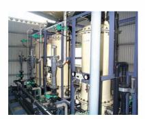
Installable with only 3000mm of ceiling height and 900mm × 1800mm of frontage even in a narrow space
