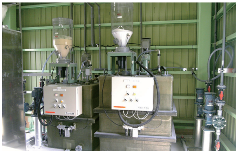
Delivery place : Tohoku region Dairy product process factory Type : Powder auto dissolver (table feeder method) Model : Y/PAD-D40F-30
