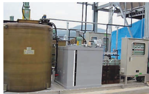
Delivery place : Kyushu region Beer manufacturer Type : Liquid polymer auto dissolver Model : L/PAD-150V+MT2000F
