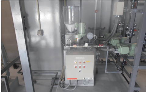
Delivery place : Tottori pref. Waste disposal site Type : Powder polymer auto dissolver Model : PAD-Q4V-15
