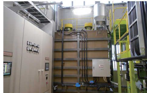
Delivery place : Okayama pref. Sludge recycling center Type : Organic conditioner dissolver Model : PAD-Q500F-400
