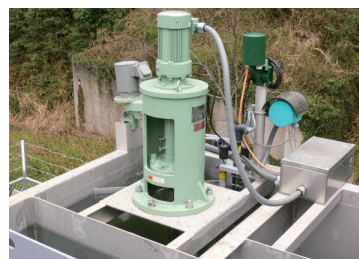
NTC type agitator Water purification plant
