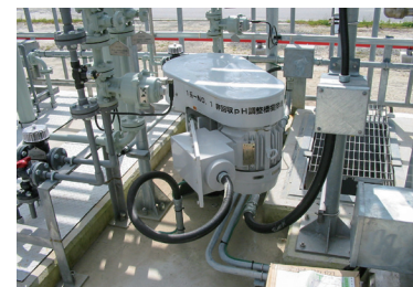
NTB type agitator Power plant
