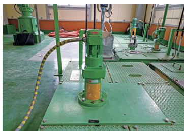
NTG type agitator Garbage disposal site
