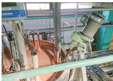
NKA type agitator Private wastewater treatment
