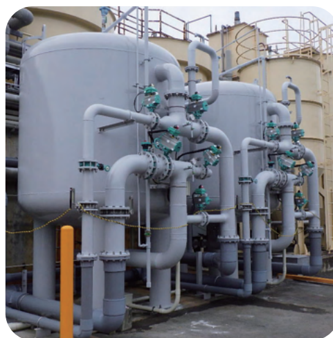
Filtration tower dimensions: ø2,900mm x SH1,830mm
